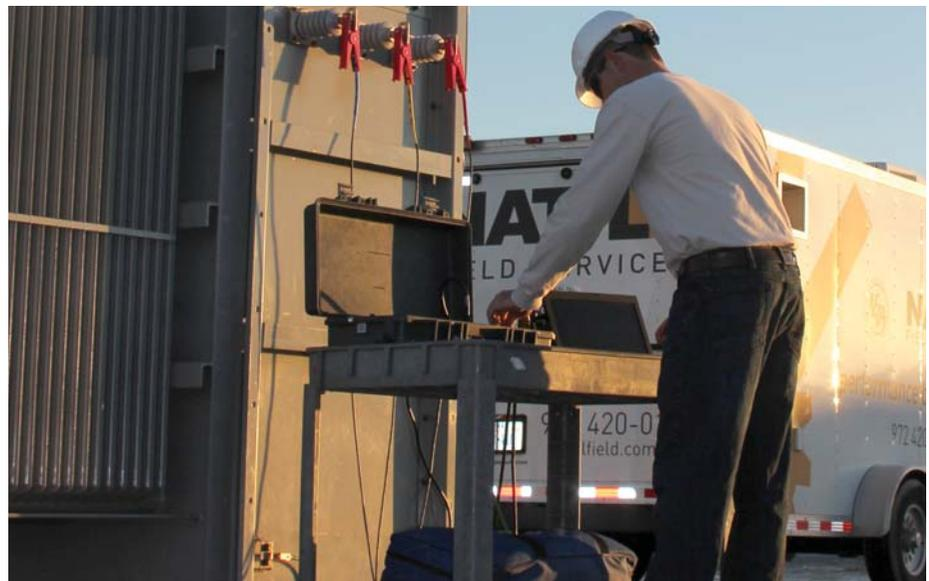
A NETA-certified ETT performs a power factor test on a de-energized 3,750kVA transformer.
